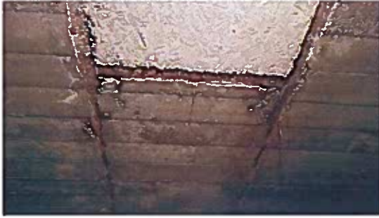
Photograph 1 ↑ Looking at concrete ceiling (and patch) located in former file storage room, in basement, where historic water intrusion events have occurred from.
